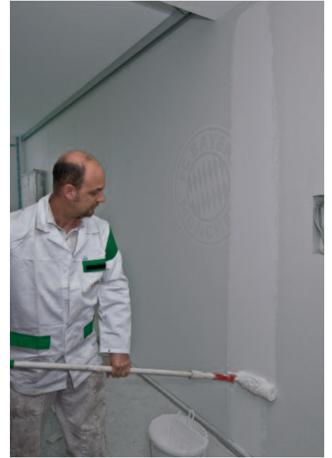
After the adhesive has thoroughly dried apply a good and even coat of paint.
